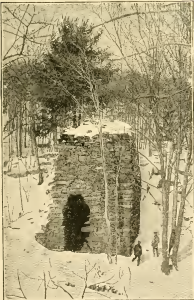
Old iron furnace, near Warwick, N. Y.
