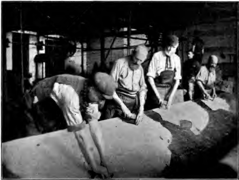
FIG. 85.—Scouring large Seal-Skins by Hand.
