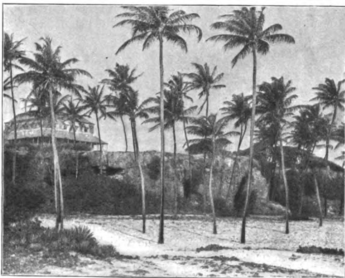
THE CRANE HOTEL, FROM THE BEACH
