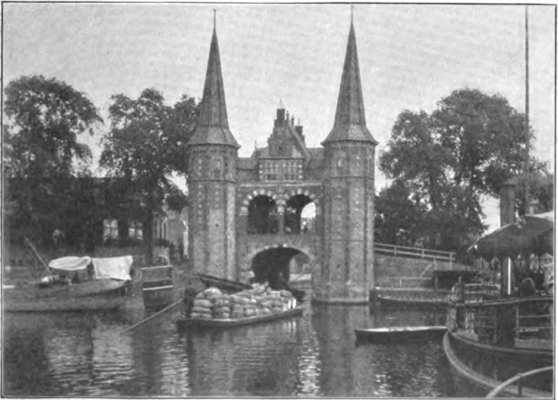
THE WATER GATE, SNEEK
