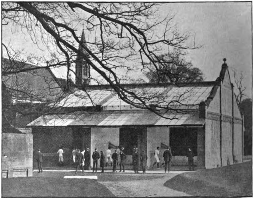
THE FIVES-COURTS AT SHREWSBURY SCHOOL, BUILT FROM PROFITS
