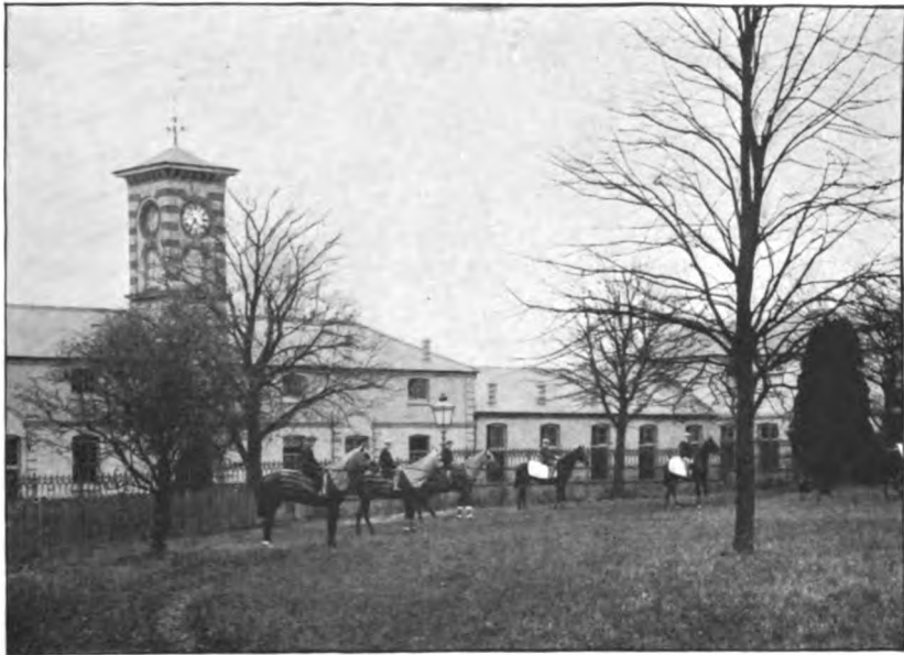
SOME OF THE STRING AT BEDFORD COTTAGE
