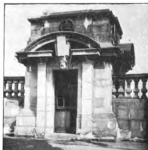
Lodge at Entrance to St. James's Park from Buckingham Palace Road
