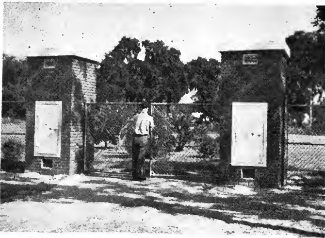
Entrance gate, typical of Jacksonville playgrounds. These piers contain electric switches and equipment.
