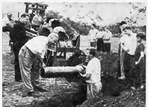
New drainage system will keep the athletic field dry.
