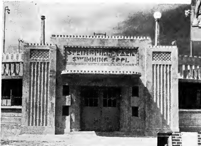
Front entrance of the Springfield Swimming Pool. The pool itself is built above ground.
