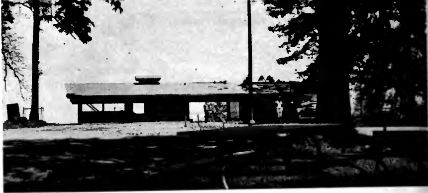
Killbuck Park concessions-service building nears completion.
