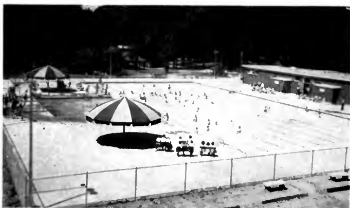
T-shaped pool, Albany, Georgia. Note bathhouse and ample sundeck. Diving area is separated from swimmers by a float line. A Charles M. Graves design.
