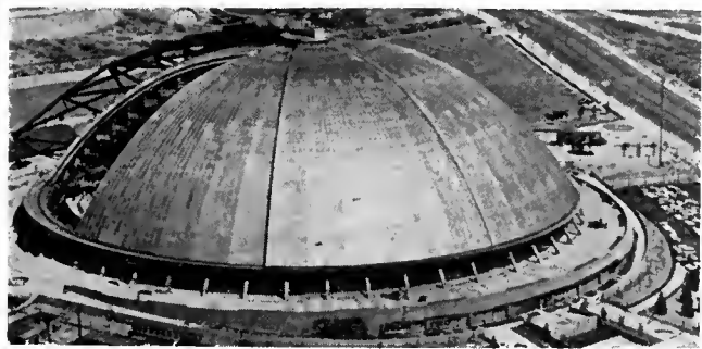
Pittsburgh's new $21,000,000 public auditorium has a retractable, stainless-steel roof which can open or shut in two-and-a-half minutes. Total capacity: 13,600. Main roof support: cantilever frame projecting 205 feet over auditorium.
