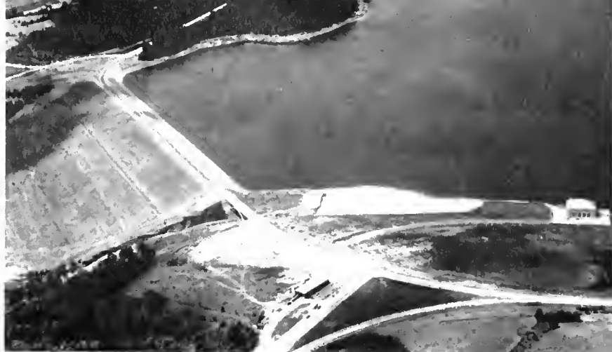
Neversink Dam on a Delaware tributary is typical of the nine large multi-purpose dams to be built in the Delaware Basin in the next thirty years.
