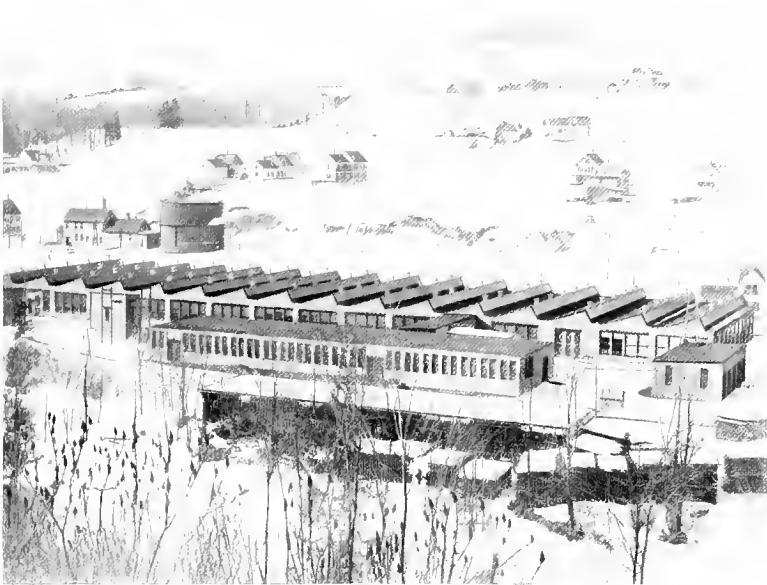
Lower Plant where Machines are Assembled
