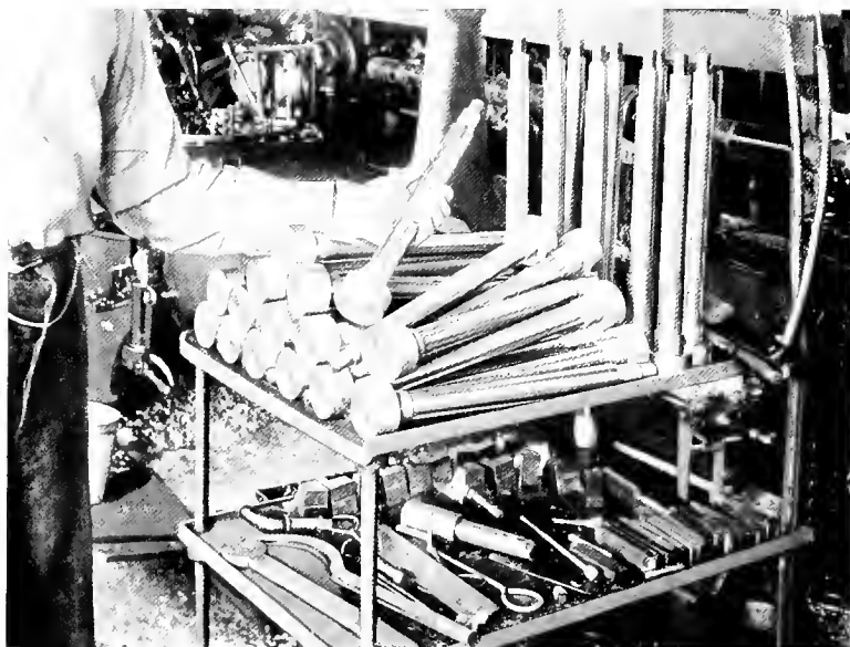
Bar Work. (Pieces made from long bar of stock)
