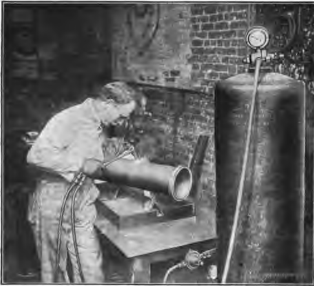
Fig. 4. Welding together the Parts of a Drawn Steel Retort. The Operator feeds the Joint with a Special Grade of Iron Wire
