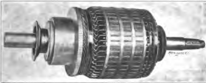
Fig. 69. The Completed Armature.
