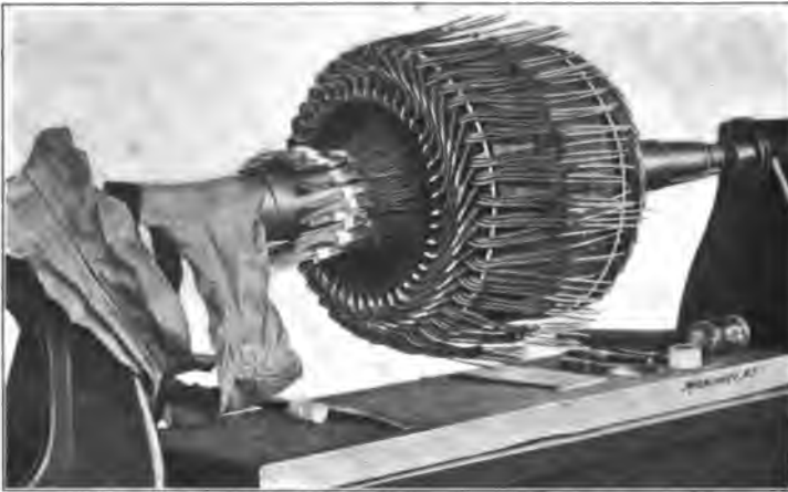
Fig. 66. Truing-up the Winding.
