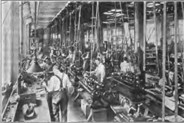
Fig. 1. A Partial View of the Tool-making Department
