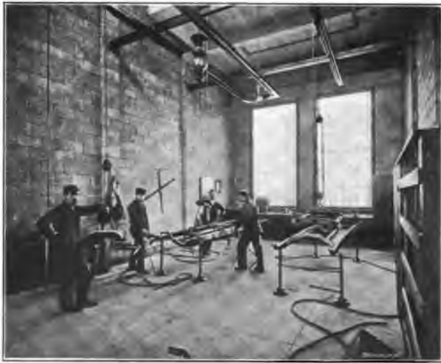
Fig. 37. Room in which the Frames are drilled and riveted by Pneumatic Tools
