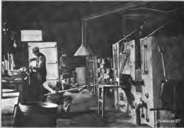
Fig. 39. Gear Case-hardening Room in the Premier Factory
