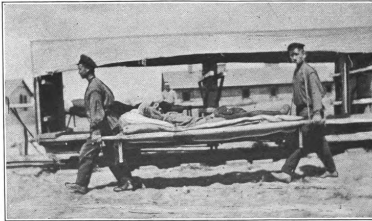
PLACING SICK ON DE CAUVILLE CAR.
