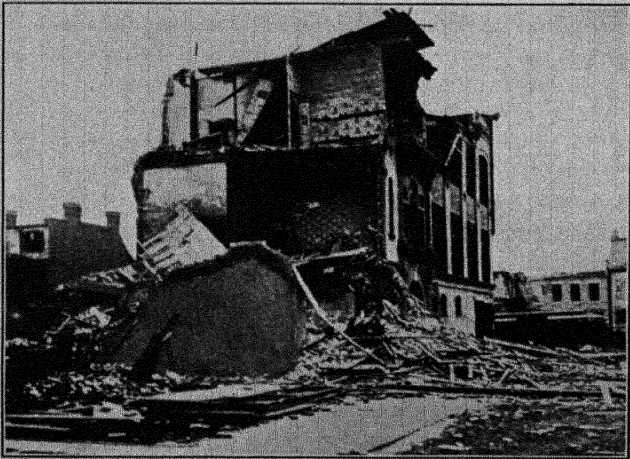
FIG. 138. — Wreckage of Anchor Hall, Jefferson and Park Avenues, St. Louis, May 27, 1896.
