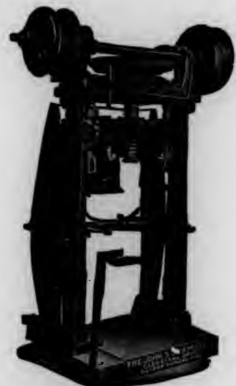
NEW "ECONOMY" (PATENTED) HEADING-UP MACHINE
