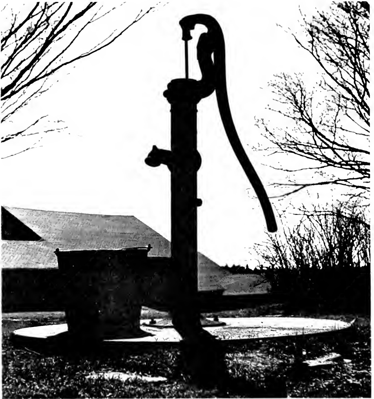
FIGURE 12— Old-fashioned lift pump.
