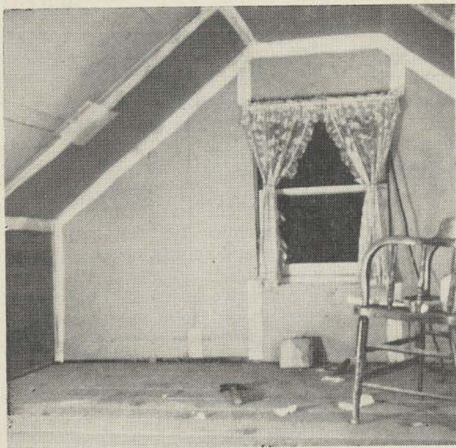
Figure 1. Walls after cardboard and muslin have been applied,
