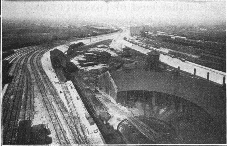
TRACK ELEVATION IN CHICAGO BY THE CHICAGO AND WESTERN INDIANA R. R. LOOKING NORTH FROM 49TH STREET.
