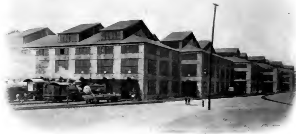
EDDYSTONE ERECTING SHOP
