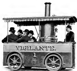
STEAM INSPECTION CAR
