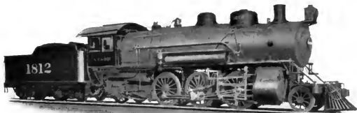
BALANCED COMPOUND PRAIRIE TYPE LOCOMOTIVE For the Atchison, Topeka and Santa Fe Railway
