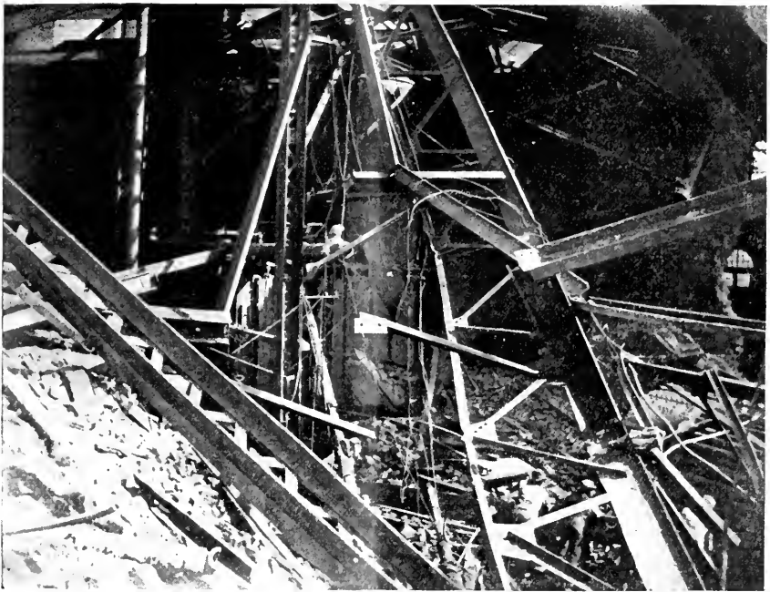
FIG. 3.— SHOWING SOME OF THE WRECKAGE IN DETAIL.
