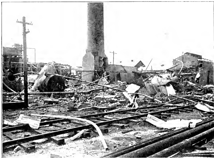
FIG. 1. WRECKED BOILER HOUSE, TEXAS CITY.
