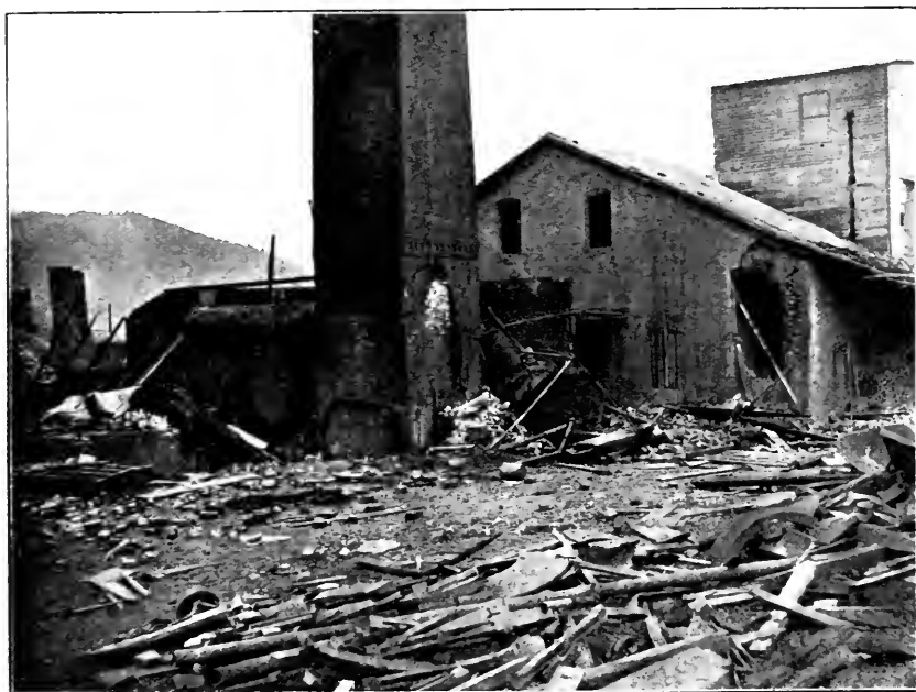
BOILER EXPLOSION AT CROW'S RUN, PA.
