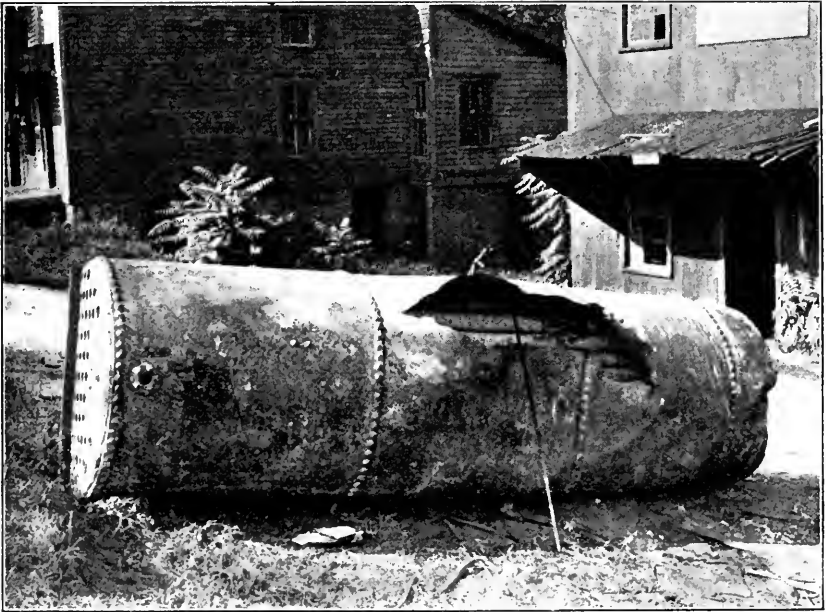
RUPTURED BOILER AT BATTLE CREEK, MICH.
