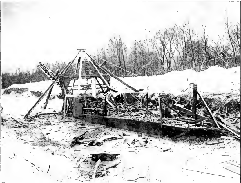
EXPLOSION OF A DREDGE BOILER, JUDICIAL DITCH NO. 51, NORMAN COUNTY, MINNESOTA.
