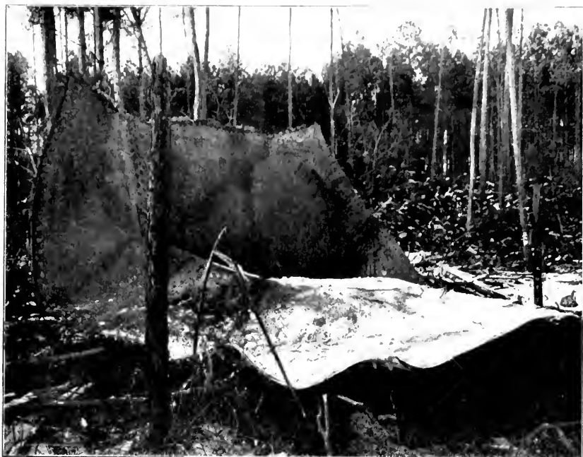
FIG. 2. SHELL PLATES OF ATHOL BOILER.
