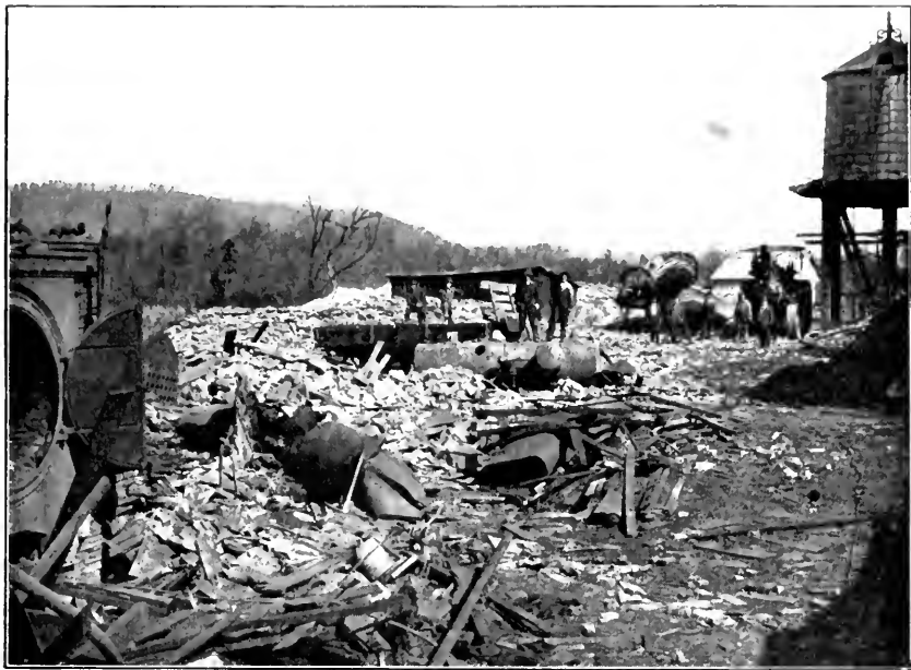
FIG. 2. SHOWING THE DESTRUCTION OF THE BOILER HOUSE AT ARRINGTON, VA.
