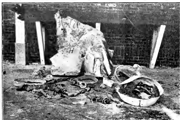
FIG. 1. EXPLODED WATER TANK. Case Eight.
