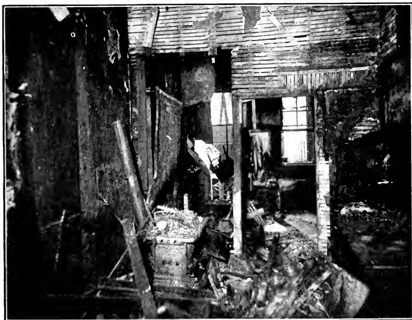
HEATING BOILER EXPLOSION, 1757 THIRD AVENUE, NEW YORK CITY.
