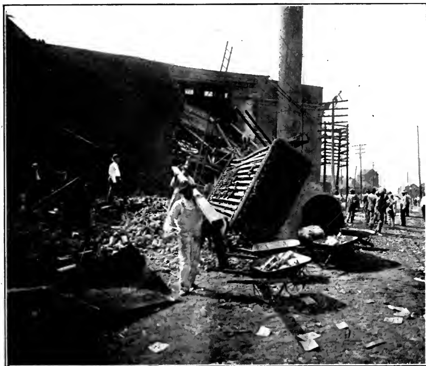
WATER TUBE BOILER EXPLOSION, MERIDIAN, MISS.
