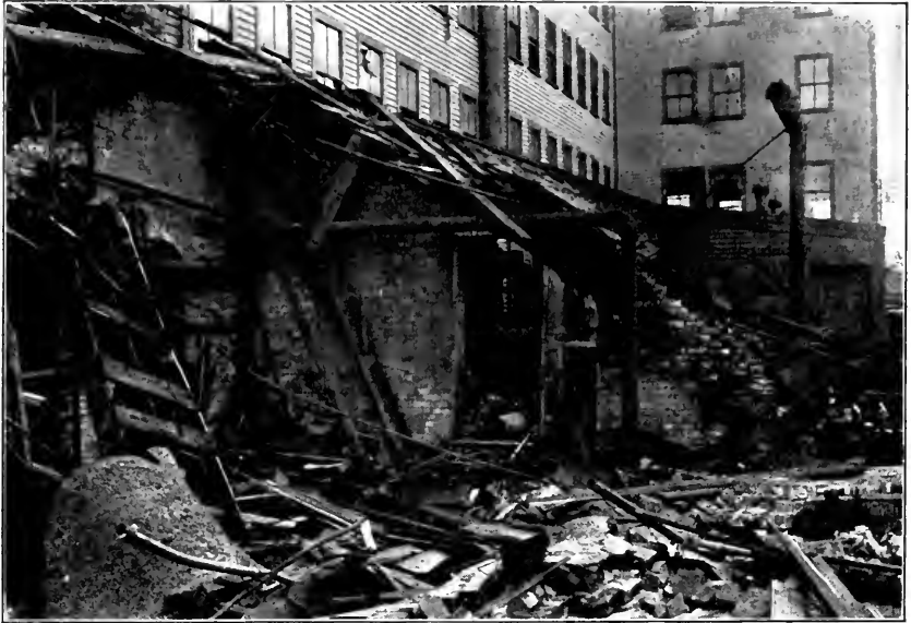
FIG. 4. WRECKED BOILER HOUSE AT EAST WEYMOUTH.
