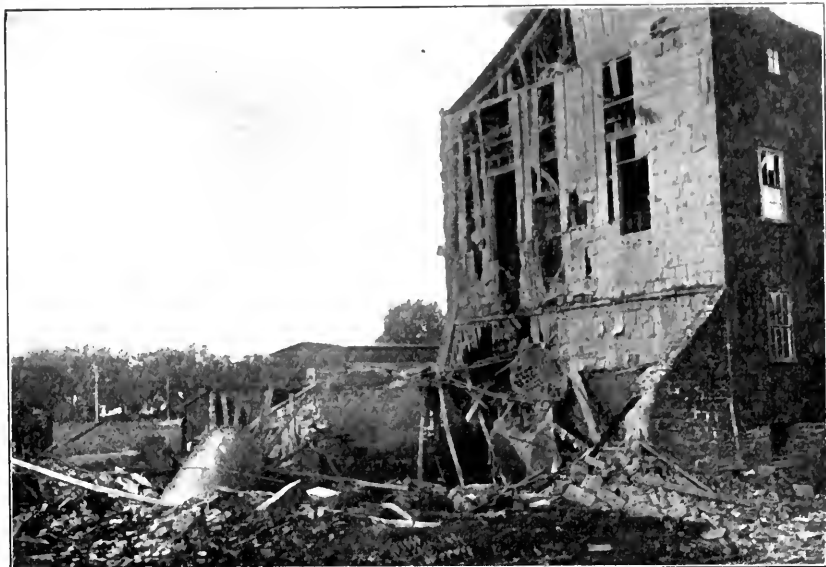
FIG. 2. WRECKED BOILER HOUSE AT COLUMBUS.
