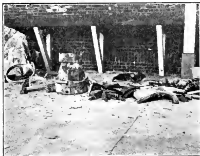
WRECK OF A SLEEPING ROOM AND OF THE HEATER. Case Eight.
