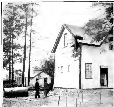
FIG. 2. BOILER'S LANDING PLACE.
