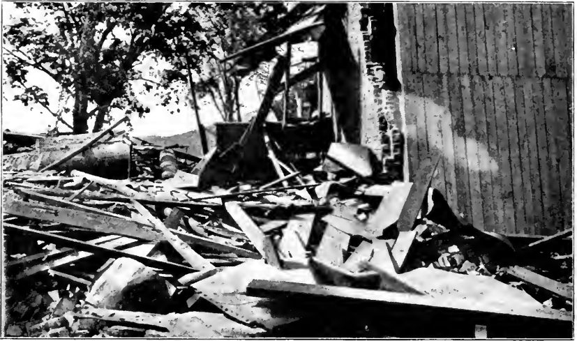
FIG. 2. DEMOLISHED BOILER HOUSE, PLEASANT VALLEY.
