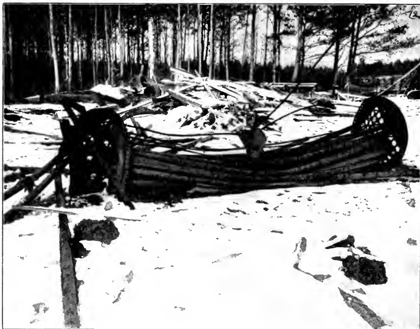
BOILER EXPLOSION, ATHOL, MD.
