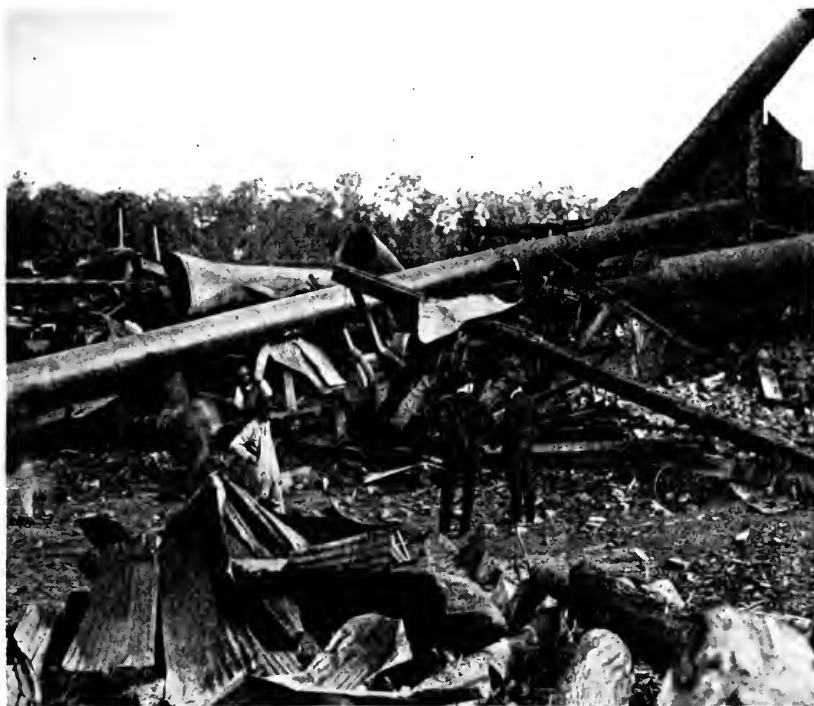
BOILER EXPLOSION AT LUMBER, SOUTH CAROLINA.
