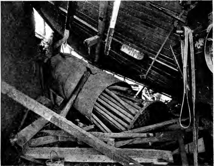
VIEW OF EXPLODED BOILER.
