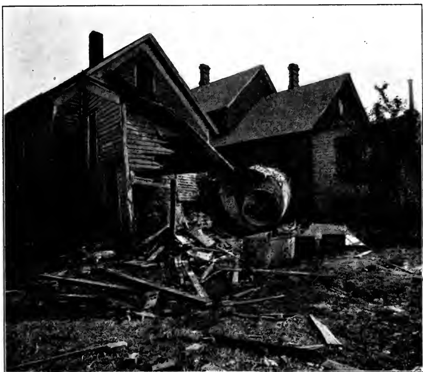
BOILER EXPLOSION AT OWOSSO, MICHIGAN.
