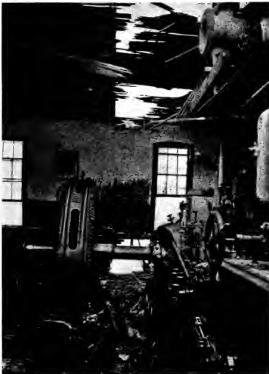
FLYWHEEL EXPLOSION. KENTUCKY UTILITIES CO.
