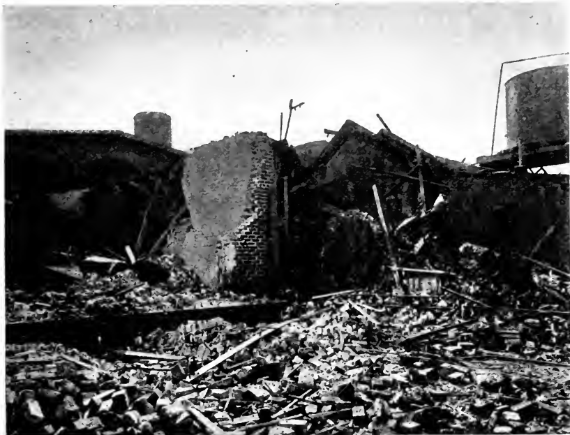
BOILER EXPLOSION AT SAVANNAH, GEORGIA.
