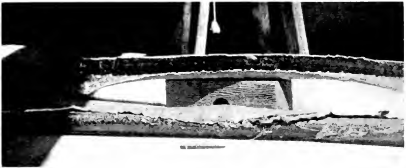
Figure 1—Cable attacked by corrosive caustics in seepage water.
