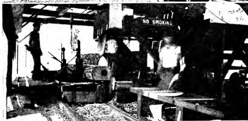
Top—The “crowning glory”—The sawmill locomotive made from parts of this and that. Center—Boiler with its open air setting and sawdust bin. Bottom—The saw carriage, showing the arrangement of two saws for extra large logs.
