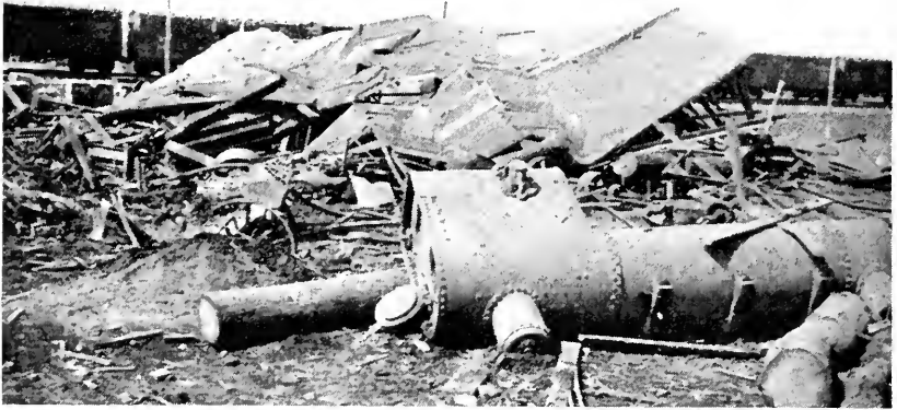
Complete destruction of a southern mill by a boiler explosion.
