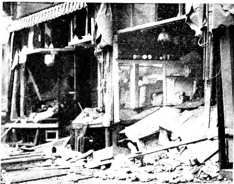
A cast iron boiler explosion on November 18, 1935, injured four persons and wrought damage estimated at $10,000 to these stores.
