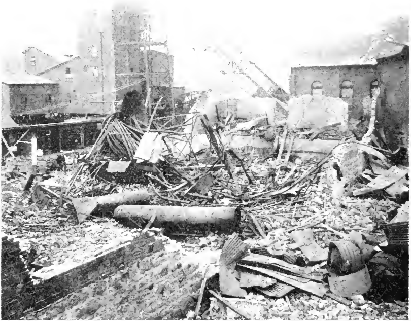
Wreckage at the mine following the boiler explosion.
