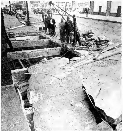
Result of ammonia explosion in cold storage warehouse.
