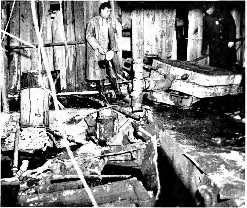
Wreckage following a heating boiler explosion at Clifton, N. J.
