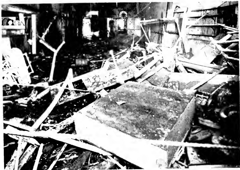
What a boiler did to its owner's dry cleaning establishment.
