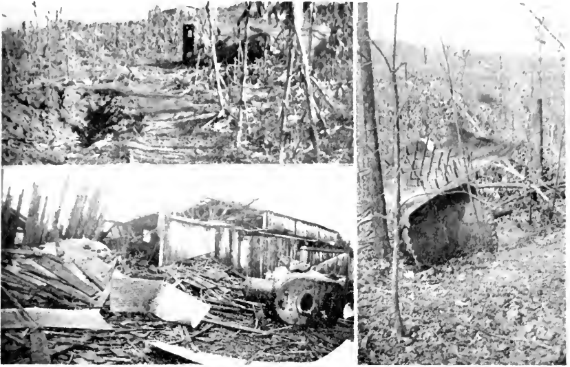
Upper left—Camden, Tennessee, boiler in a cornfield 300 ft from its setting; the hole at the left shows where the shell first landed. Lower left—results of an explosion in a Hohenwald, Tennessee, sawmill. Right—found two days after its explosion in a Powellsville, Ohio, sawmill. This part of the boiler traveled over a hill near the plant.
