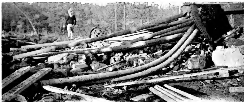
Parts of mine boiler following its explosion.
