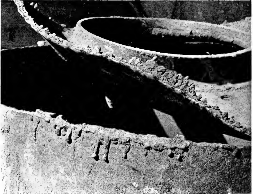
Close-up view of welded seam failure.
