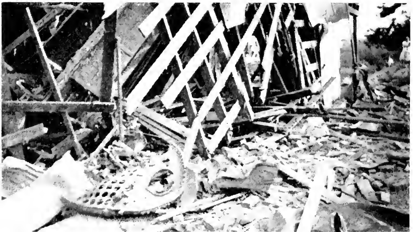
Above—Middle and rear courses of Neal, Georgia, boiler. Below—Where eight were killed in cotton gin boiler explosion.
