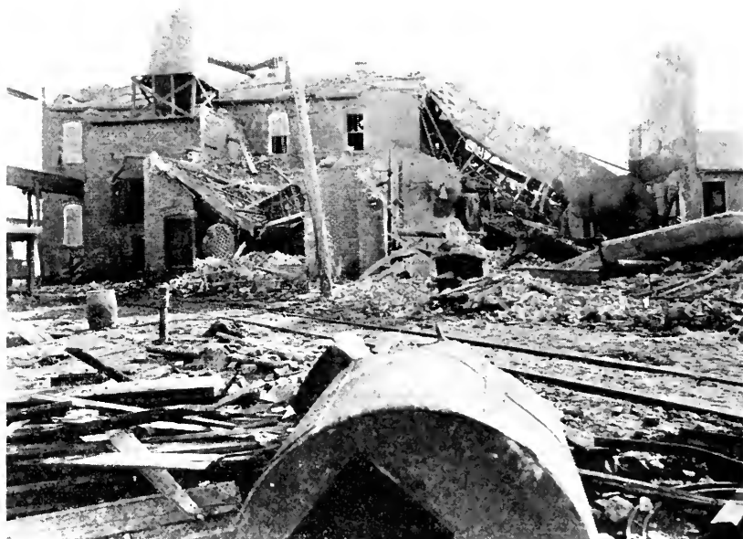
Wreckage at Hertford, North Carolina. A one-story boiler room formerly stood at the right just beyond the tracks at about the spot where the steel smokestack is lying. Near the left center of the mill building is No. 1 boiler beneath which is the engine. On the roof of the mill building at the extreme left is the rear course of the No. 2 boiler which exploded. The breeching is in the foreground.
