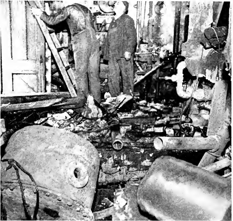
Result of cast iron blow-off tank explosion.
