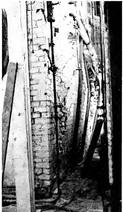
View of right side wall of No. 2 boiler showing the damaged setting. The boiler is 72" in diameter and 16' long of the horizontal return tubular type.
