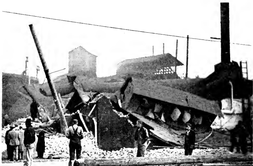
Result of external corrosion of a blank head in a bent tube type boiler.
