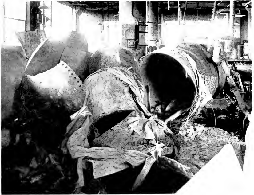
Figure 1. Remains of the vulcanizer after its explosion.
