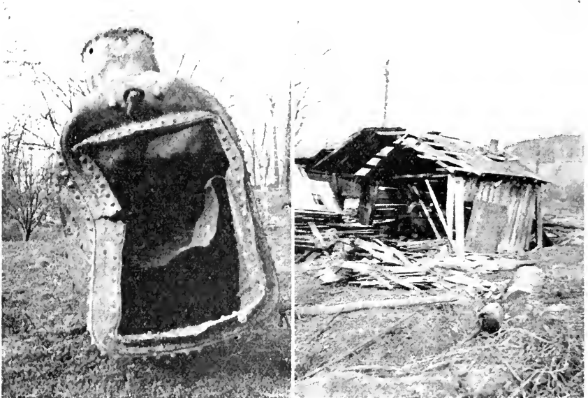
Left:—Boiler after 300 ft. journey. Right:—The shattered engine house where the eight persons who were killed or injured had gathered.
