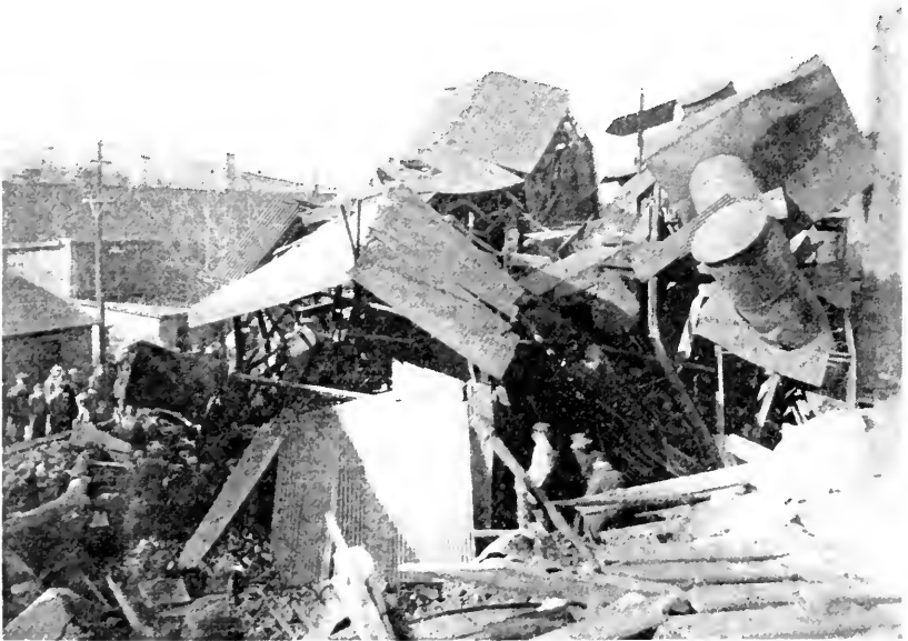
After a corroded mud drum head blew out at an Indiana paper mill.
