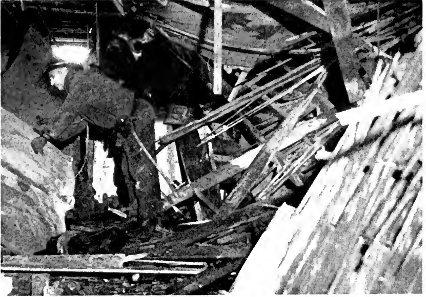
Debris inside apartment following the accident.
