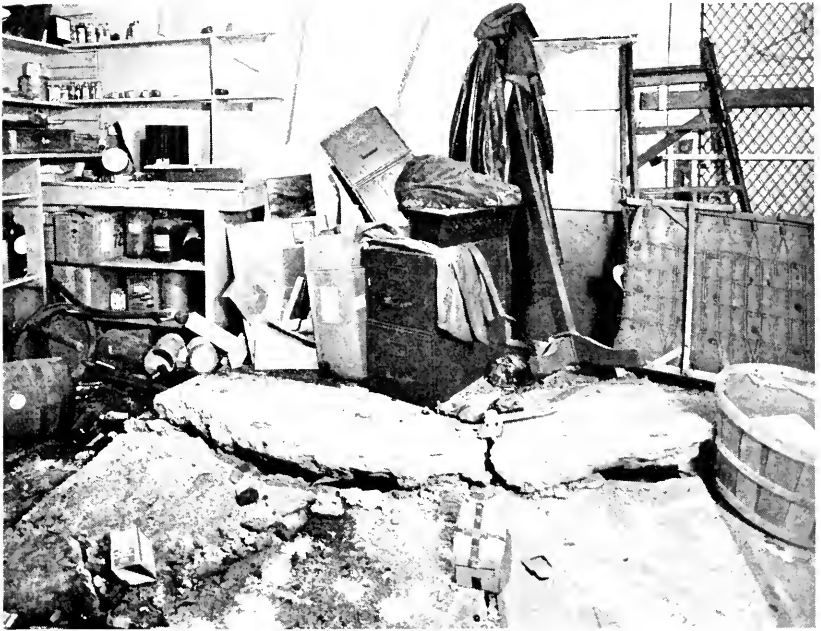
Part of drug store floor damaged by hot water heater blast.
