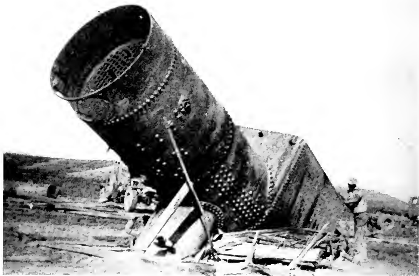
After the crown sheet pulled off its stays.
