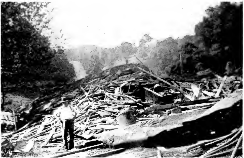
After a sawmill boiler explosion in West Virginia. The scene is typical of wreckage following this type of accident.
