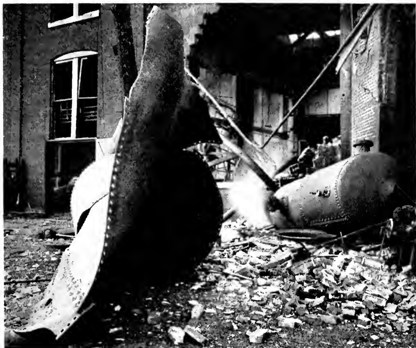
Following the ignition of lubricating oil vapor.
