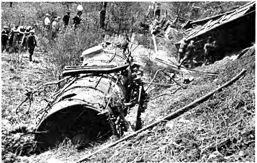
Main shell of locomotive after explosion which probably was caused by low water.
