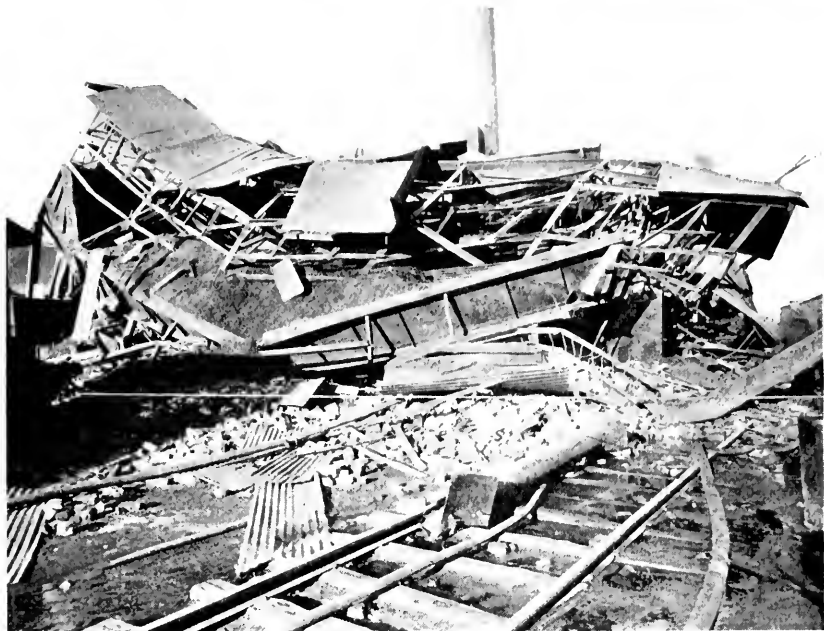
A bunker of coal collapses into the debris to complicate the search for a fireman's body.
