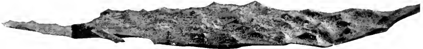
Figure 3. Extreme corrosion of boiler plate, the cause of an explosion that badly wrecked a mill and damaged property of four other owners.
