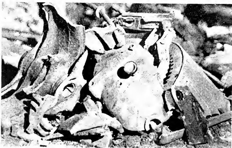
Parts of the boilers which were picked up after the accident. The boiler, which was one year old, was not insured.
