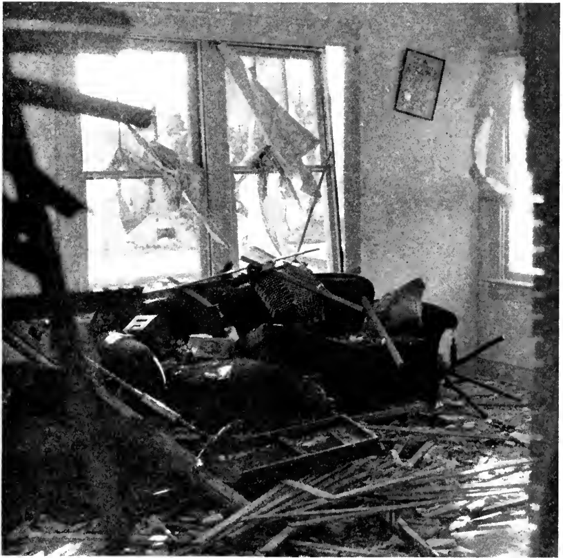
Home wrecked by bursting of hot water tank.
