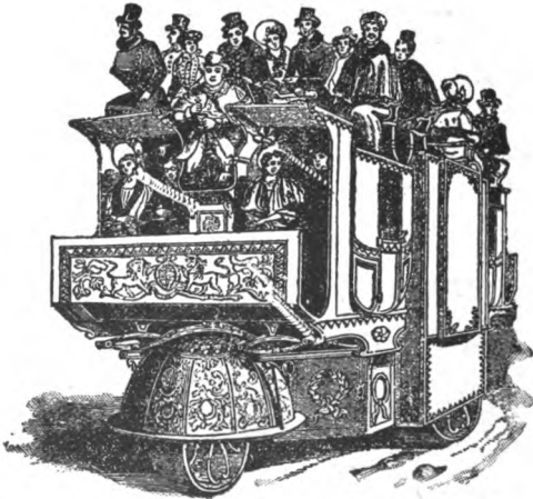
Church's steam locomotive for highways. 1832.
