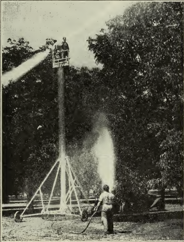
Fig. 16.—A tower for spraying large walnut trees, built after Plan No. C-145 (see footnote 8, p. 22). Note the position of the outrigger wheels when the tower is in use.
