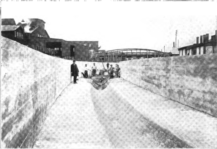
Large Concrete Sewer in Aramingo Canal.
