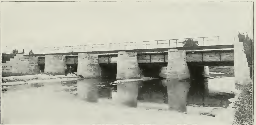
View of Completed Aqueduct.
