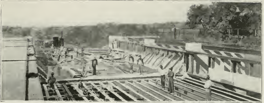
Depositing Concrete for Lining of Aqueduct No. 7.
