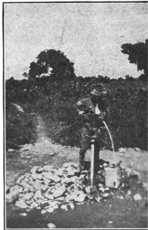
FIG. 109.—Tube well.
