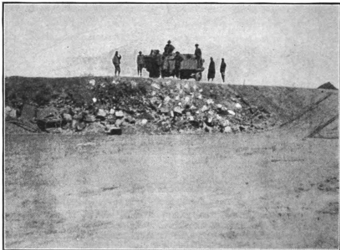
FIG. 106.—Rubbish dump. The only exposed rubbish is along the advancing margin of the pile. The top of the dump is entirely covered over and smooth. ( Lewis and Miller. )
