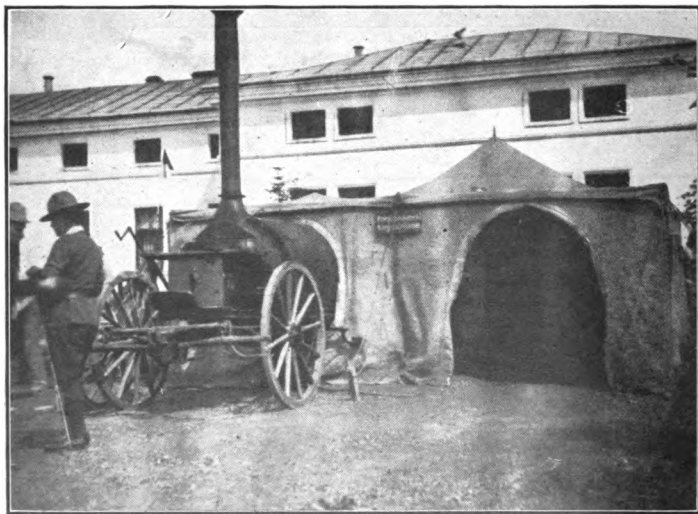
FIG. 35.—Wheeled field oven (Austrian) with tent.
