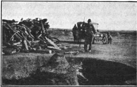
FIG. 107.—Cake tin or cone incinerator.
