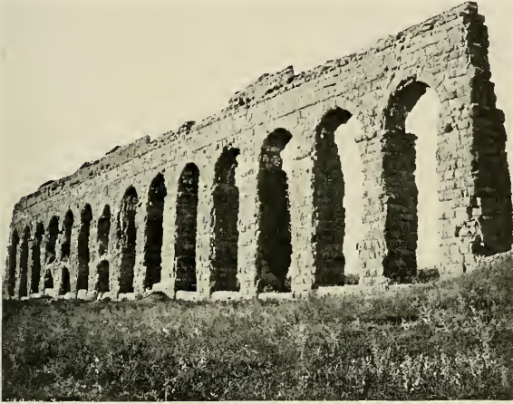
Near View of the Claudia Aqueduct
