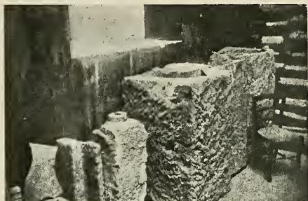
Roman Water Pipes made of Bored-out Blocks of Stone
