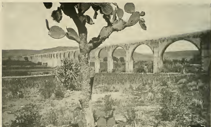
Distant View of Zempoala Aqueduct, Queretaro, Mexico
