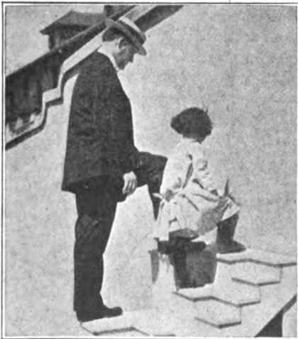
Fig. 13.—Man ascending fourteen-inch step. The child a seven-inch step. The angle at the knee is the same. In practice we make the three-foot child take the same step as the six-foot man.
