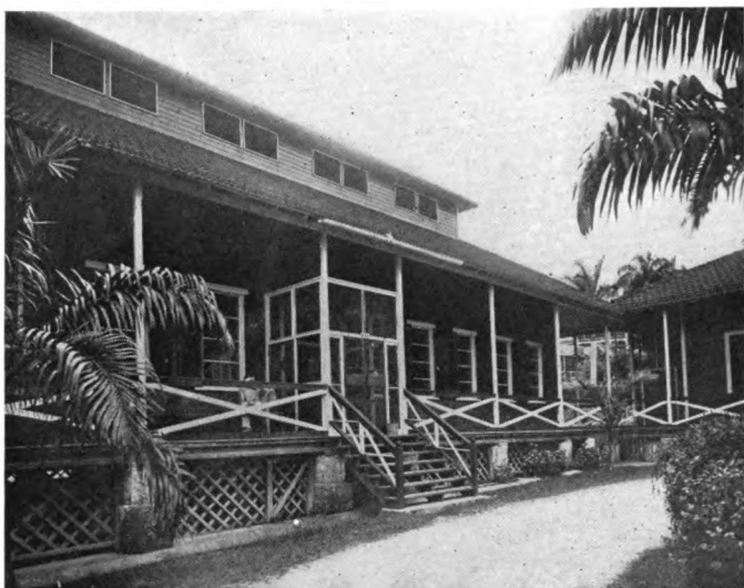
Screened Yellow-fever Ward. Ancon Hospital, Panama.
