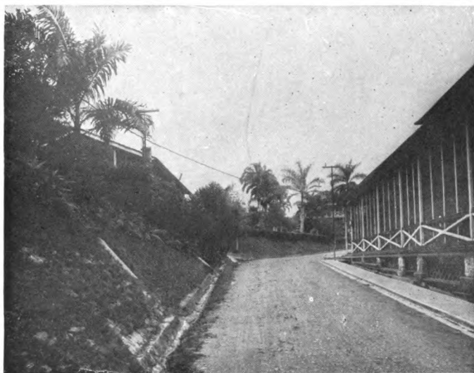
St. Charles Ward, Ancon Hospital. Building in Which Twelve Hundred Frenchmen Died of Yellow Fever.
