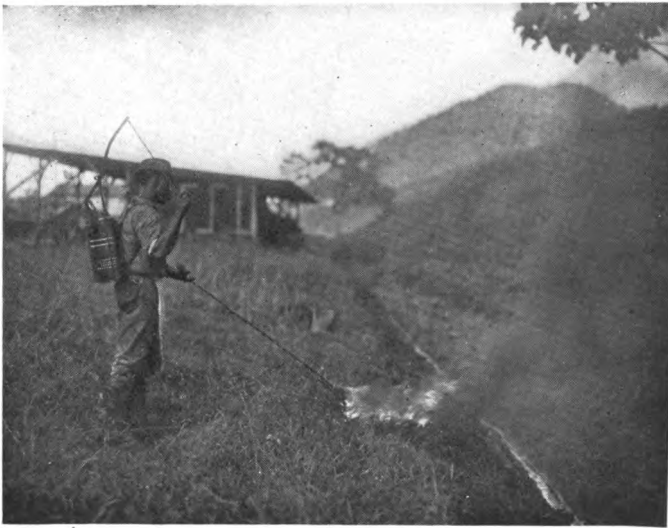
Burning Out Ditch With Oil Spray.
