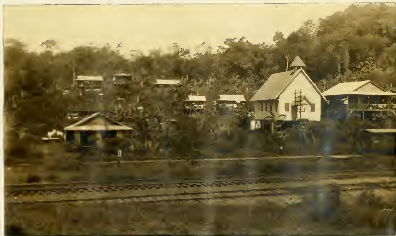
Views of Frijoles from the Sanitary Office.
