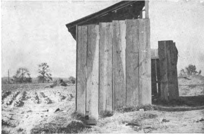
OPEN PRIVY OVER A SMALL STREAM WHICH OVERFLOWS ON A STRAWBERRY BED
