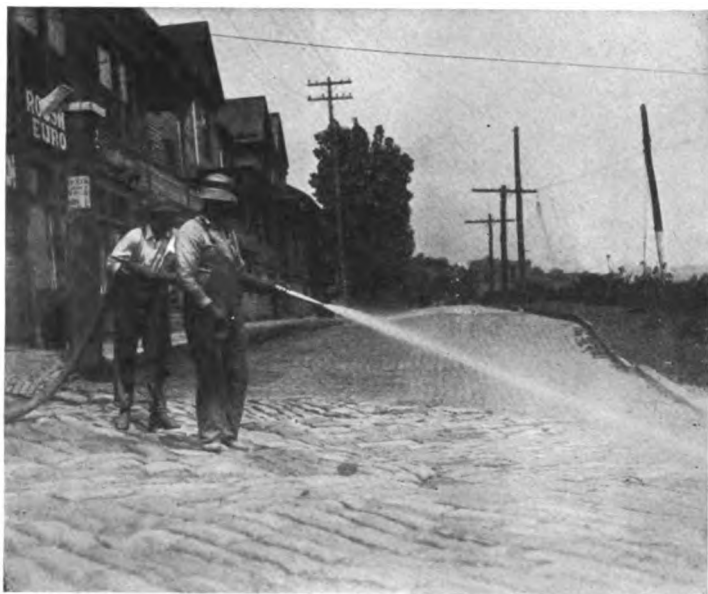
STREET FLUSHING BY HAND IS EFFECTIVE AND OFTEN CHEAP
