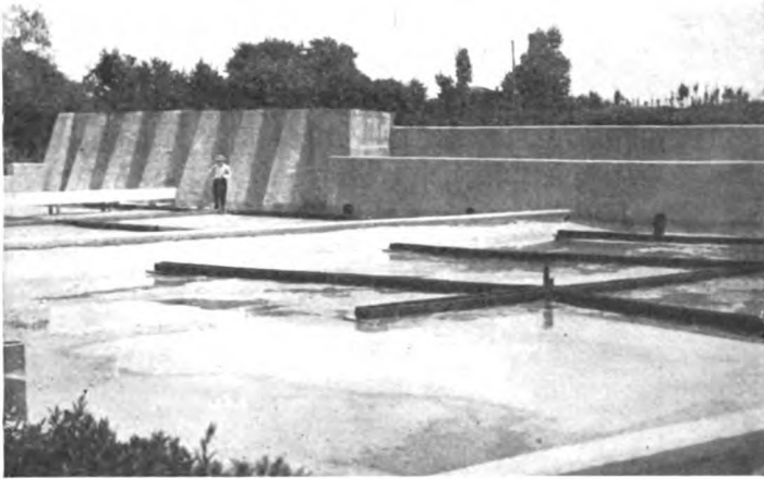
SAND BEDS FOR SEWAGE FILTRATION Liquefying tank in the distance
