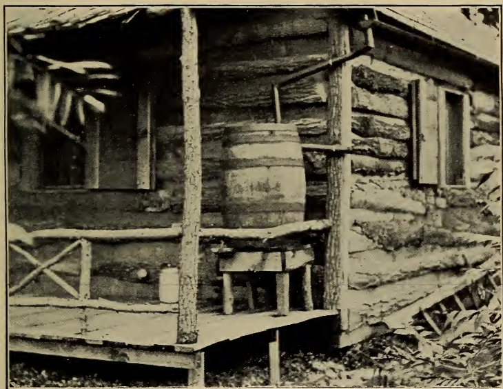
FIG. 9.—AN INEXPENSIVE AND SANITARY METHOD FOR COLLECTING RAIN-WATER. (From "Sanitation of a Country House.")
