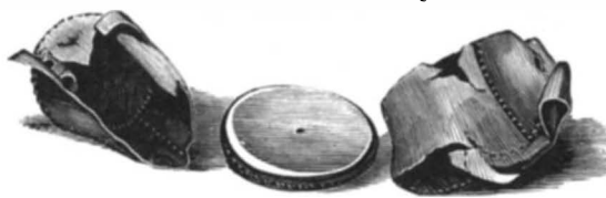
FRAGMENTS OF THE EXPLODED BOILER.
