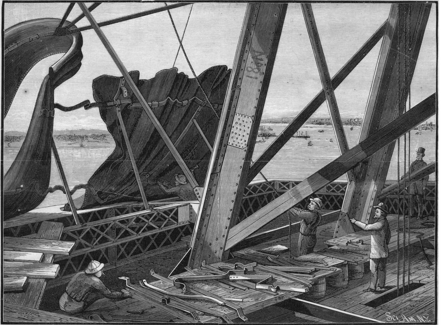
STATUE OF LIBERTY.—VIEW AT TOP OF PEDESTAL, SHOWING THE SHELL AND BRACING.
