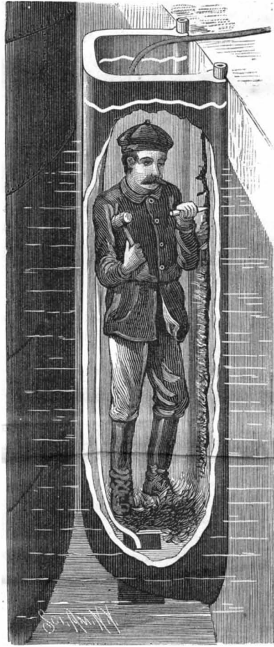
BOTTOM SECTION OF COFFER DAM AGAINST TANK WALL.
