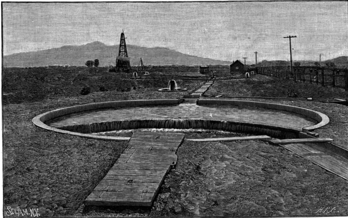
ARTESIAN WELLS AND RESERVOIR, RIVERSIDE, CAL.
