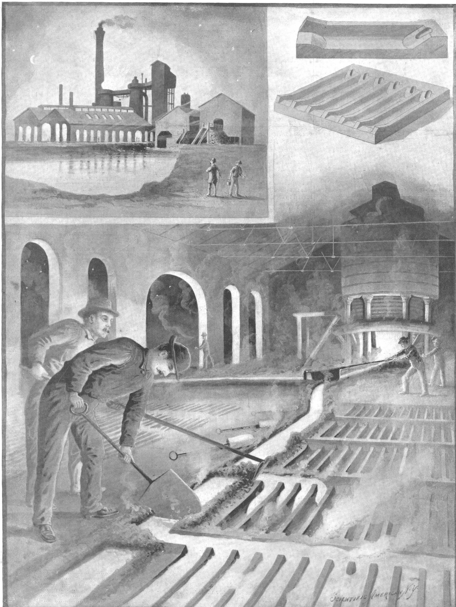
THE "ALICE" FURNACE, BIRMINGHAM, ALABAMA.—[See page 391.]
