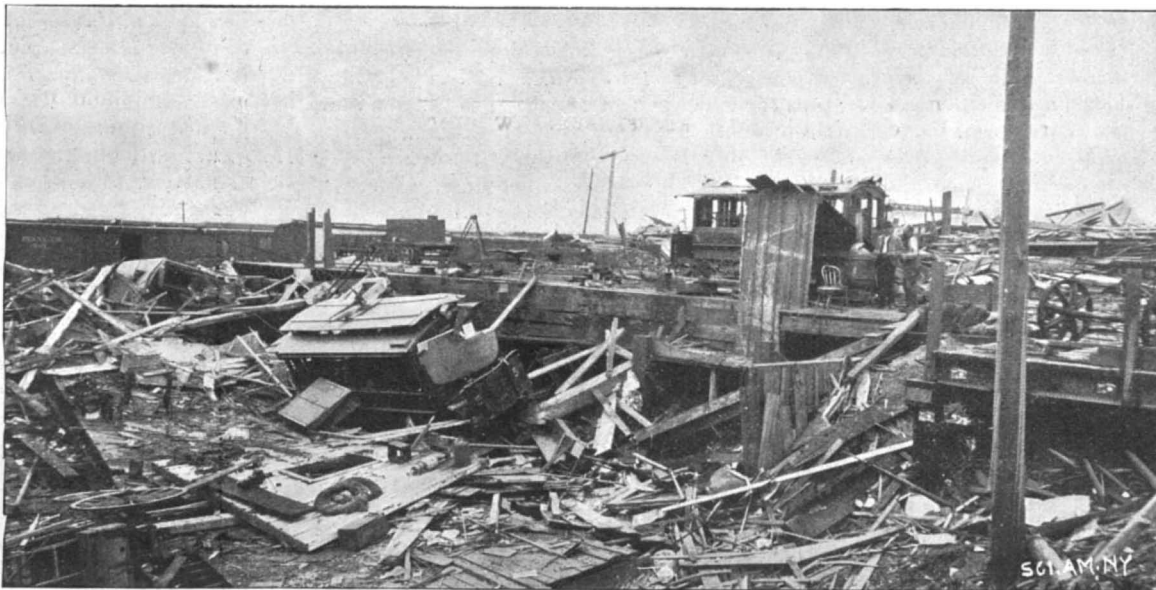
DESTRUCTION CAUSED BY LATERAL FORCE OF WIND.
