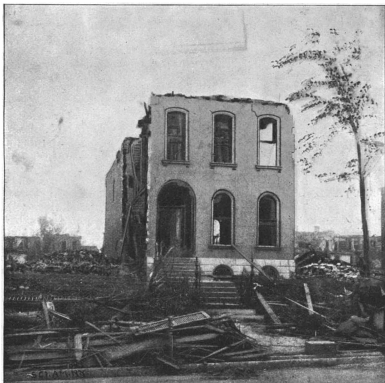
HOUSE SHOWING BOTH WALLS BLOWN OUT UPON APPROACH OF THE VACUUM AREA.
