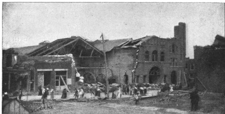
RAILWAY POWER HOUSE AFTER THE STORM.
