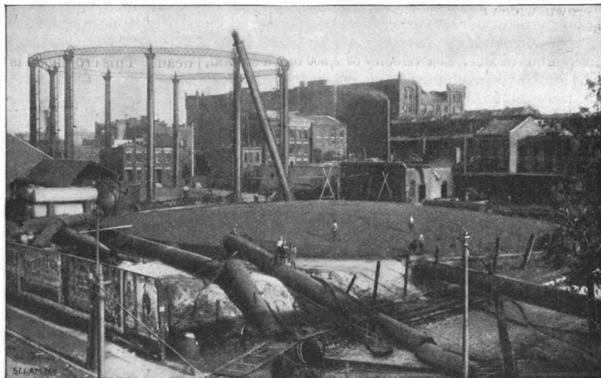
DESTRUCTION OF GAS TANK AT FOURTEENTH AND GRATIOT STREETS.
