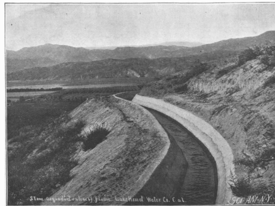
THE AQUEDUCT-IRRIGATED LANDS IN THE VALLEY BELOW.
