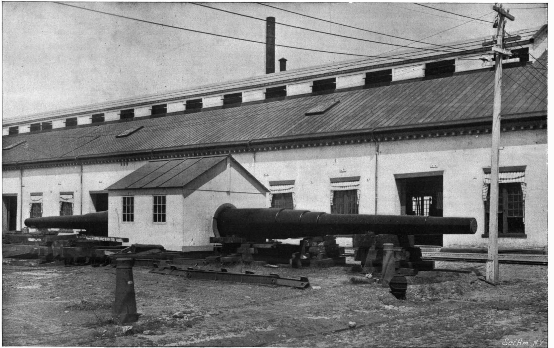
FINISHED GUN PROVIDED WITH TEMPORARY SHOP.
