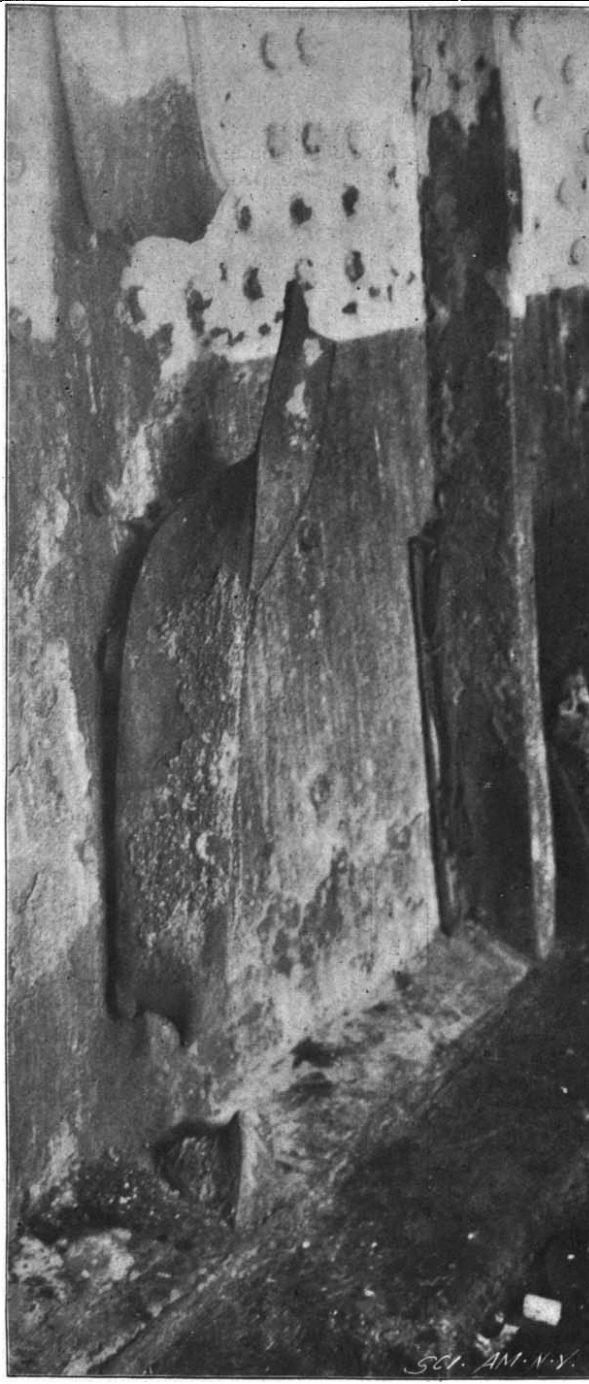
7.—Starboard Ship's Frame on Gun Deck Cut in Two Places by Fragments of 6-inch Shell.
