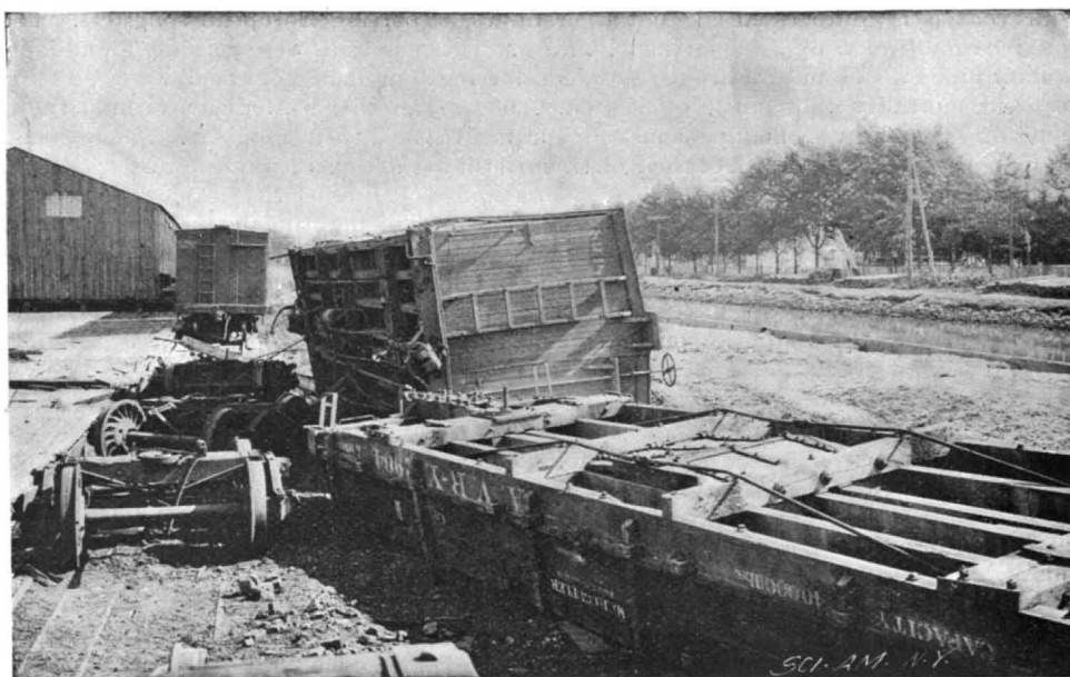
FREIGHT CARS WRECKED BY A TORNADO AT TONAWANDA, N. Y.
