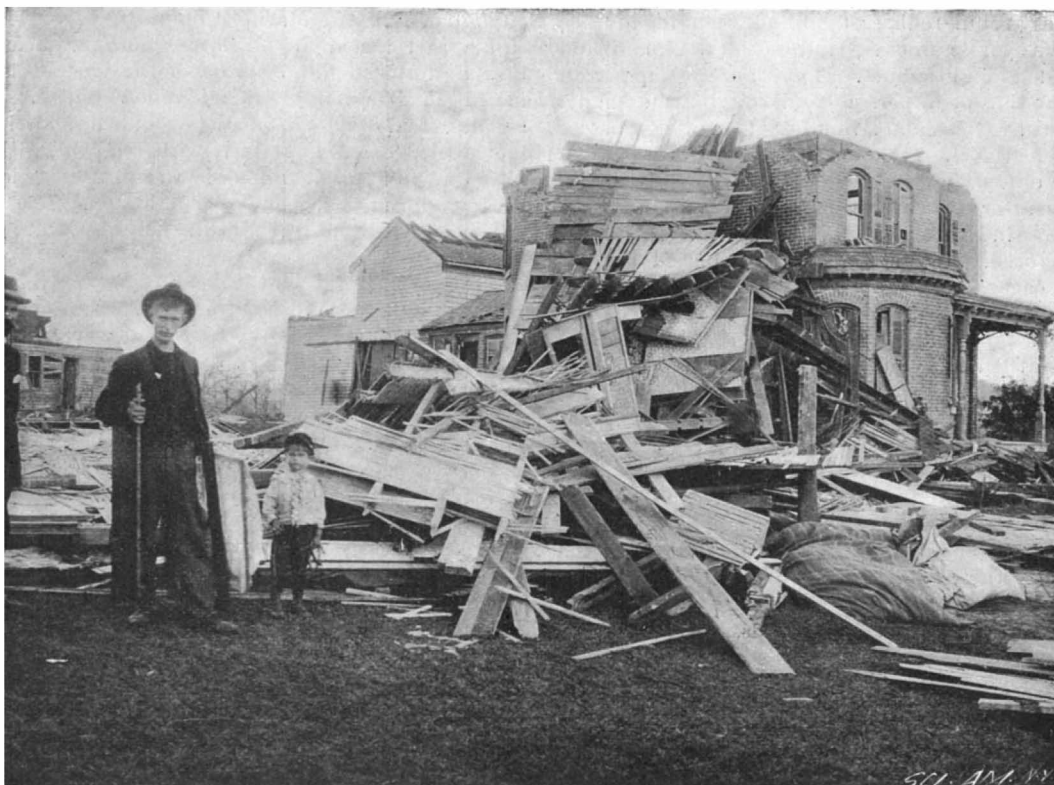
HOUSE COMPLETELY WRECKED BY A CYCLONE AT MERRITTON, CANADA.
