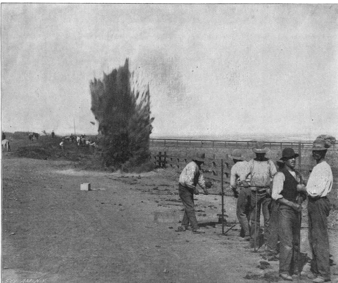
BLASTING IN HARD GROUND; FROM AN INSTANTANEOUS PHOTOGRAPH.
