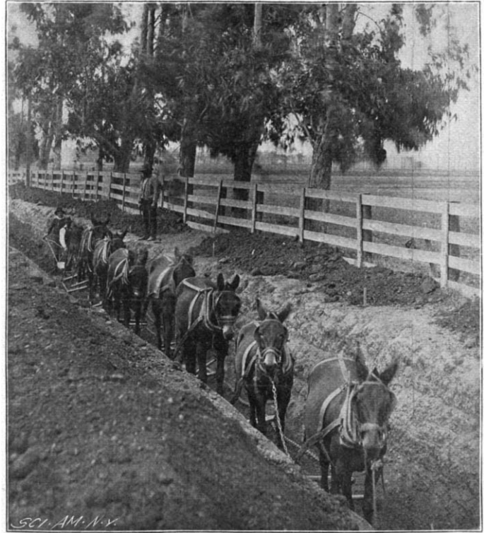
DIGGING PIPE-DITCH WITH PLOW AND MULES NEAR SAN MATEO.
