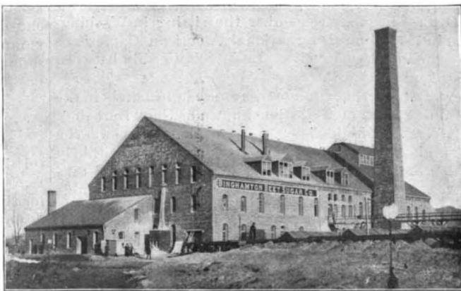
General View of the Exterior of the Building.
