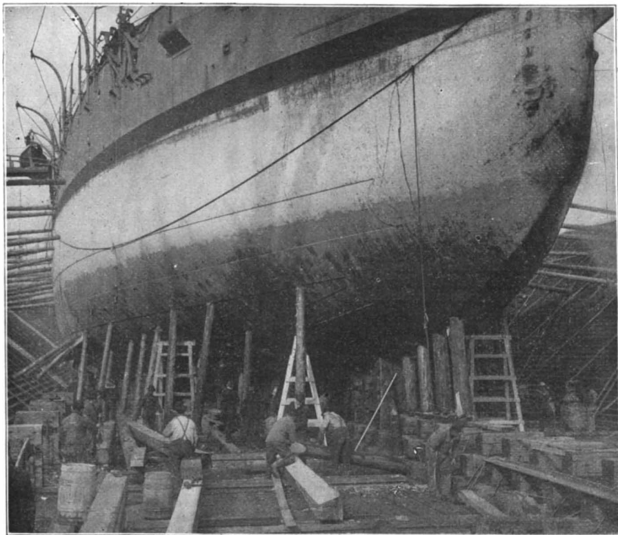
5.—Bow View of Ship when Water was First Pumped Out of Dock, Showing Method of Shoring.
