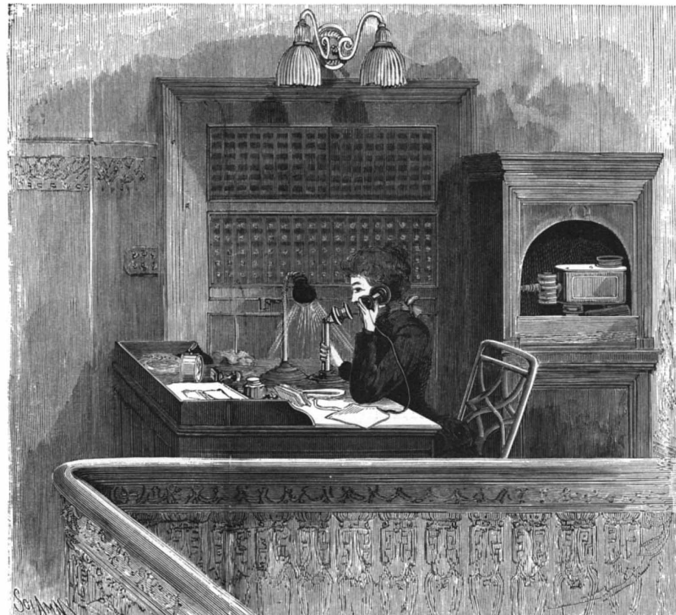
Local Floor Station.
