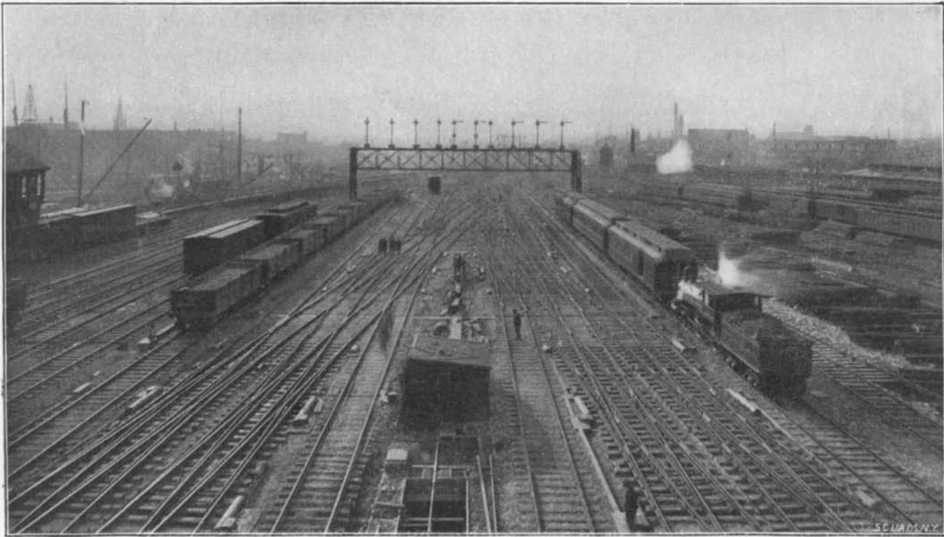
1.—SOUTH BOSTON TERMINAL YARD, SHOWING DIAMOND CROSSINGS AND SWITCHES, AND ONE OF THE SIGNAL BRIDGES.
